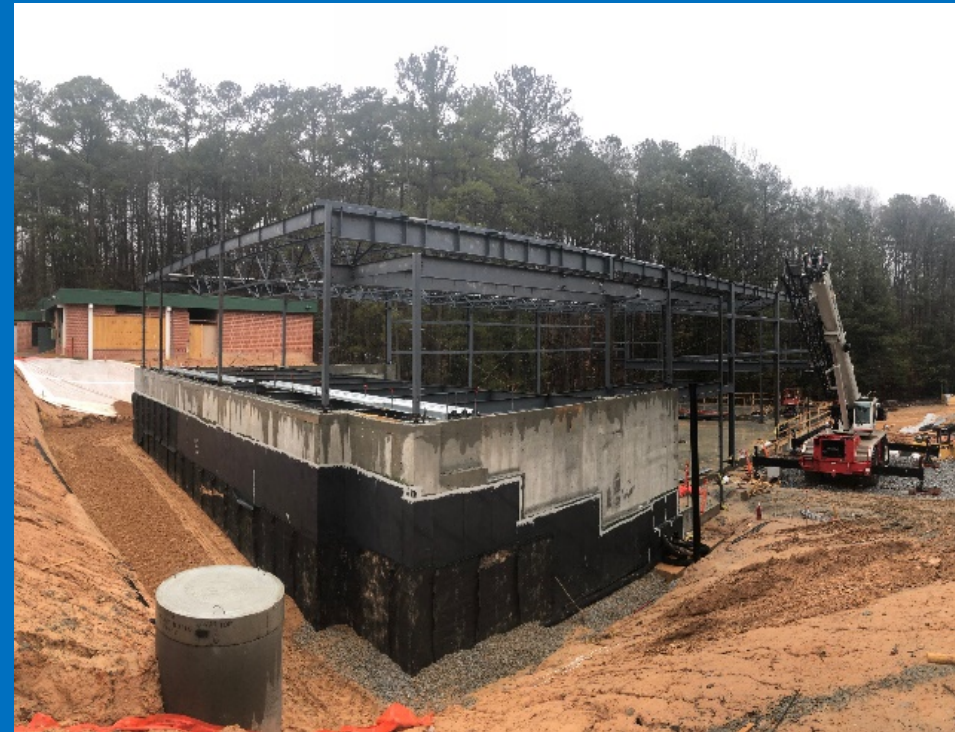
Gymnasium Steel Erection
