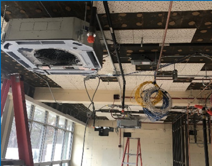
SW Wing VRF Cassette Installation
