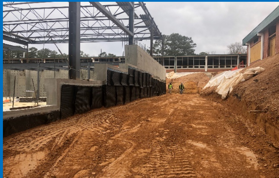
Foundation Wall Backfill Ongoing
