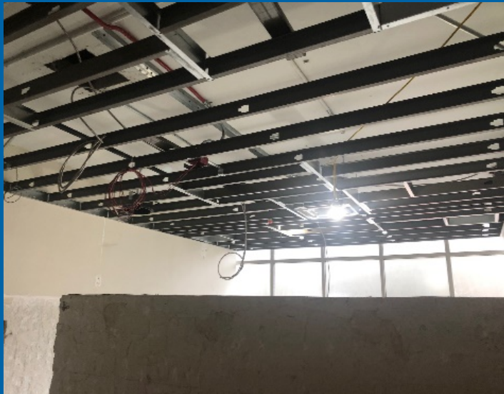
SW Wing Hard Ceiling Ready for Cover-Up Inspections
