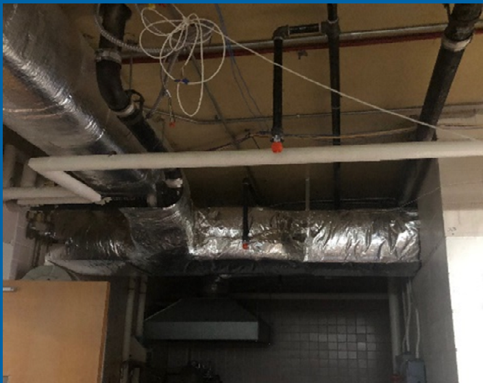
Duct Insulation and Fire Protection at Kitchen/Cafeteria
